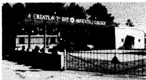
Church House in Guys, TN, 2006
